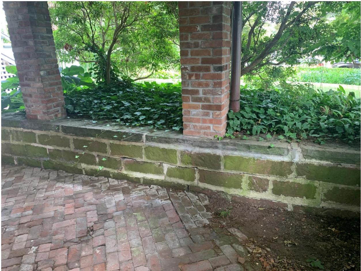
Figure 25. Retaining Wall Condition at basement patio
